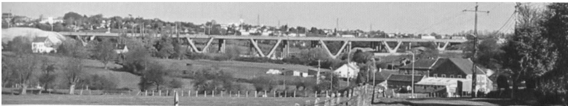
Figure 3: Continuous high speed railway viaduct with V-shape supports
